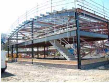
A new building site undergoing consultation with Angus Council Building Standards
